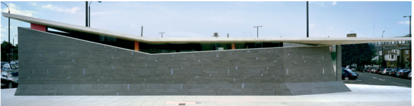
The long elevation of the building; from this angle, the purpose of the structure is unknowable.
