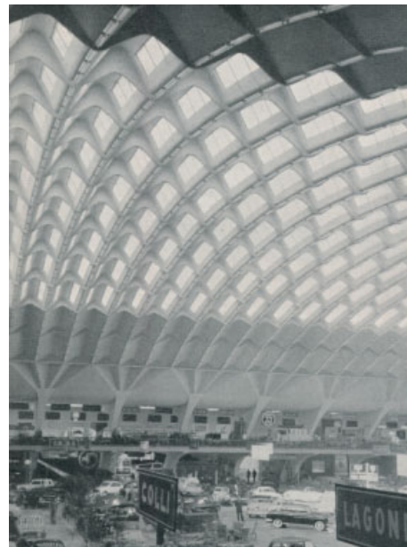
Pier Luigi Nervi, Exhibition Hall, Turin, Italy, 1949 The long span vaults were constructed using prefabricated ferro-cement panels to reduce on-site formwork.
