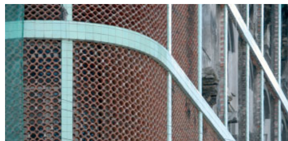
The Cobogó is a facade element that is assembled into a screenwall thus providing ventilation and shading. One of its most radical applications can be seen in Recife in Brazil, in the application of a second building envelope constructed around an existing building, the Luciano Costa House, an eclectic building from the 1910s that was redesigned in 1959 by the architect Delfim Amorim.
