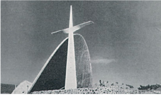
Felix Candela, Lomas de Cuernavaca Church, Mexico, 1959 A double-curved saddle roof developed from a hyperbolic surface to create an opening nearly 22 metres (72 feet) in height.
