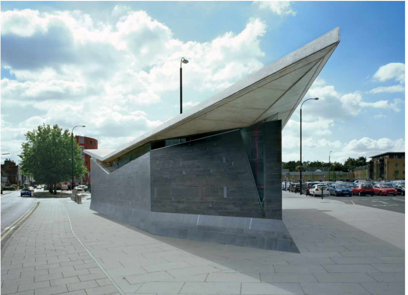
The concrete roof is given an edge detail that creates a line of shadow, reinforcing the angularity of the structure – a detail inspired by the work of Carlo Scarpa.
