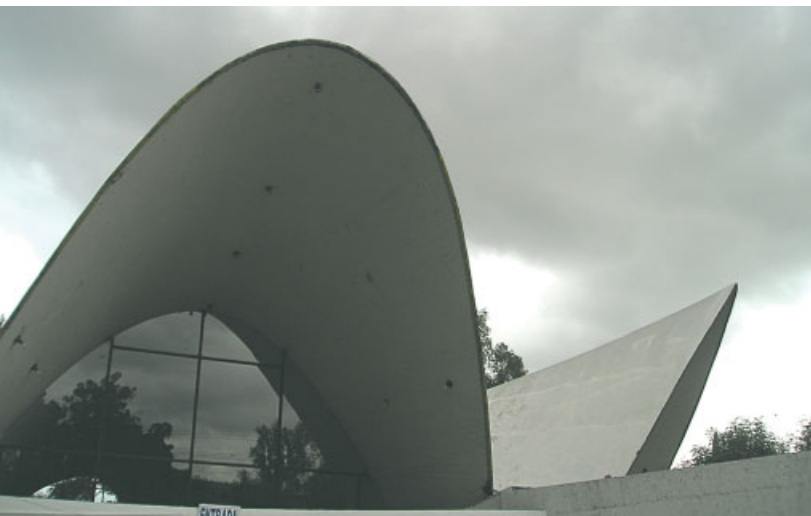
Felix Candela, Los Manantiales restaurant, Xochimilco, Mexico, 1958 The geometry here developed from a series of interconnected hyperbolic surfaces. The thinness of the concrete shell is expressed in the elevations.
