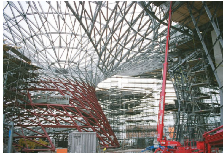
Complex roof structure of the BMW Welt building in Munich by Coop Himmelb(l)au architects and Bollinger + Grohmann structural engineers. See 'Form, Force, Performance: Multi-Parametric Structural Design' on page 20.
