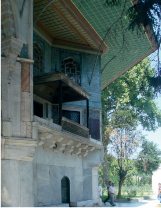
The Revan Kiosk in the Topkapi palace in Istanbul, Turkey, shows passive cooling strategies similar to the vernacular example in Abyaneh in Iran. The deep open recess on the first floor acts as a shade for the two-storey-high facade. The door on the first floor is shaded by a smaller roof that shades the lower area at lower sun-angles, and accelerates the airflow to and from the interior depending on wind direction.
