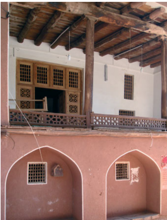
This traditional building in the famous historic village of Abyaneh, one of the oldest in Iran, is made from the typical red clay of the region. The elevation shows a number of passive environmental modulation strategies: the use of thick clay walls, with deep setbacks on the ground floor to shade window areas, and on the first floor shaded by a wide overhanging roof. All openings have simple screenwalls that enable ventilation while protecting the interior from visual penetration. In this vernacular example, building elements and spatial arrangements operate in synergy and are probably complemented by the migratory pattern of habitation in response to temperature changes at different times of the day and different seasons.
