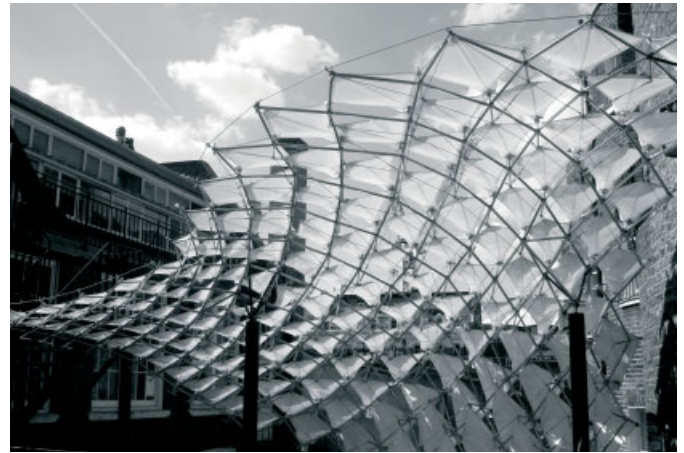
The Membrane Array Canopy, designed and constructed by the Emergent Technologies and Design masters programme in collaboration with structural engineers Buro Happold in 2007 at the Architectural Association, provides a porous canopy that allows views and substantially reduces of horizontal loads while providing shade and protection from rain.
