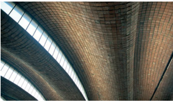
Eladio Dieste, ADF Wool Warehouse, Juanicó, Uruguay, 1994 Dieste's Gaussian vaults deliver a succinct appearance to the exterior of his designs (top), while resulting in spaces of extraordinary beauty and well-regulated light conditions in the interior (bottom).
