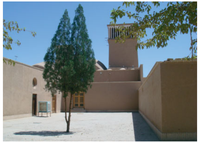
View of a courtyard of traditional residences in Yazd, Iran. The climate is very dry with cold winters and hot summers. The temperature can fluctuate dramatically between night and day and summer and winter. Temperatures of 40°C (104°F) in the summer and -20°C (-68°F) in the winter have been recorded. The city of Yazd is especially well known for its historical architecture, which is uniquely adapted to its desert surroundings. Several passive thermal modulation strategies are simultaneously present in this courtyard setting: the thick brick walls, limited openings towards the perimeter, the tree in the centre, the wind tower, domed roofs and air vents on top of the domes (partly obscured by the tree in the centre). However, these features are in stark contrast to the air-conditioning unit on the left-hand side of the court that renders several of the passive strategies redundant. Performative capacity and passive environmental modulation strategies of such traditional architecture are in this way often obliterated and replaced by energy-consuming electrical devices that have become status symbols in many parts of the world.
