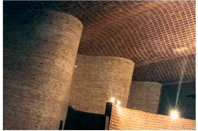
Eladio Dieste, The Church of Jesus Christ the Worker, Atlántida, Uruguay, 1960 Both the walls and the roof are double-curved surfaces, and the intersection of these shows Dieste's mastery of construction techniques.
